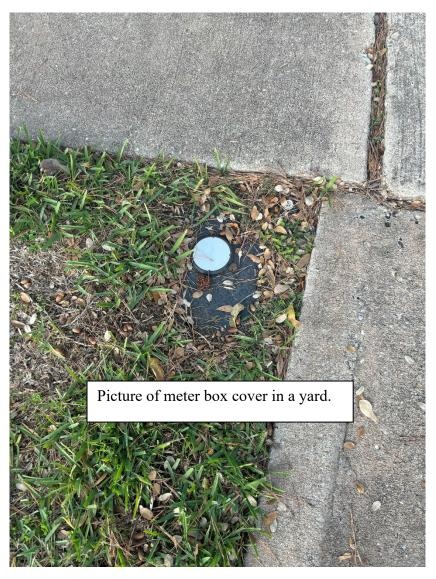
When you open your meter box there may be dirt covering the meter register. You can remove the dirt by hand and flip the lid of the register open. (Note: Do not use shovels in the meter box as this could damage the register or break the water pipe.)
